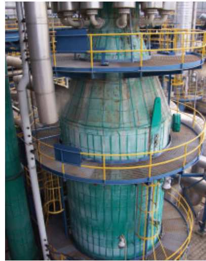
Reactor Vessel 1 prior to fibre installation
