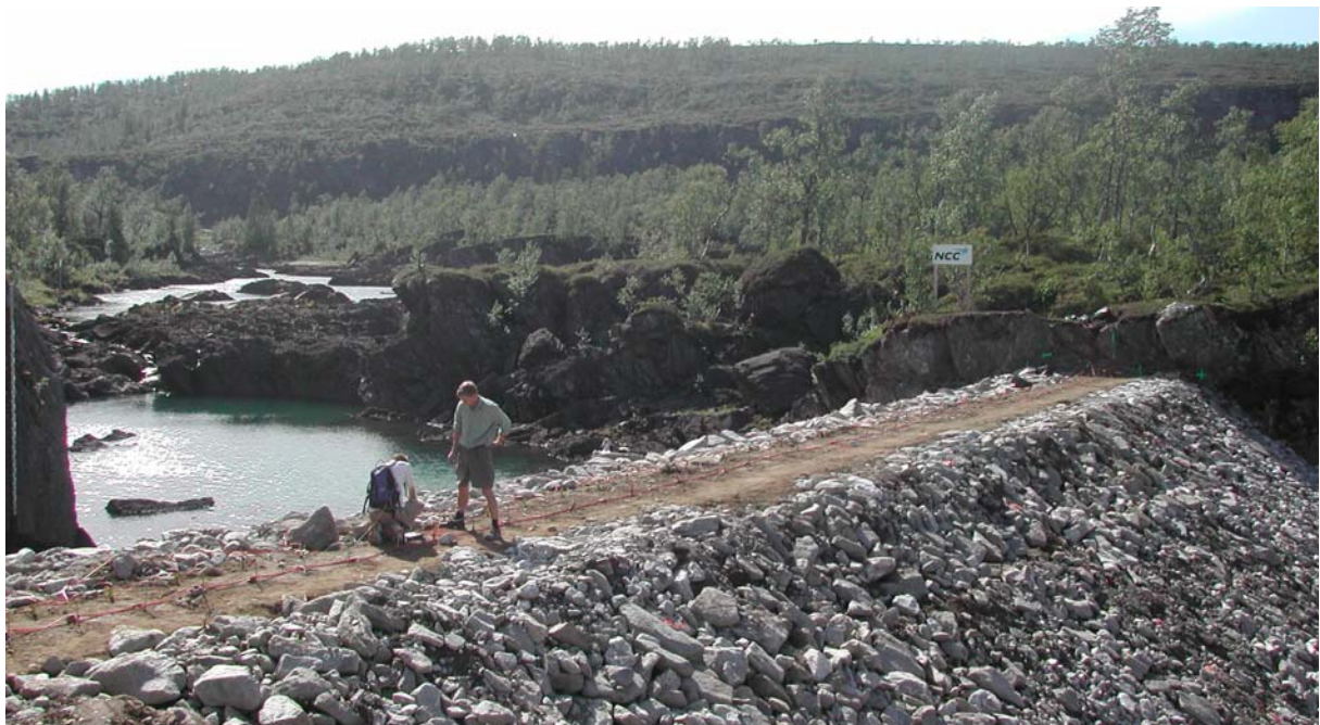
Figure 14 Downstream view of the dam at low reservoir level.
