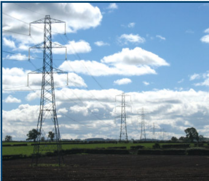
Testing the integrity of overhead fibre wrapped around power cables
