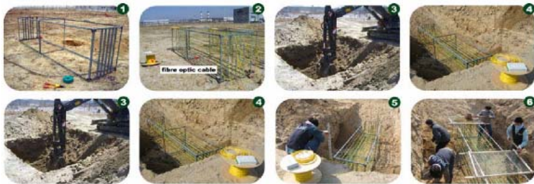
■ Installation procedure at the testing site
