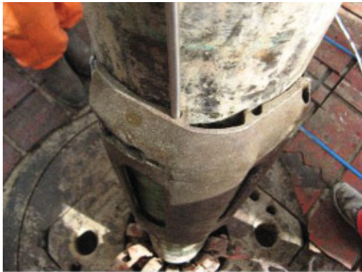
Sensing cable attached to the outside of 7" casing with a metal cross-coupling protector
